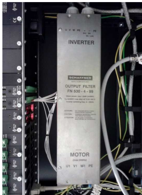
Figure 6-22. Schaffner FN-530-4-99 LC filter installed in the control cubicle.
